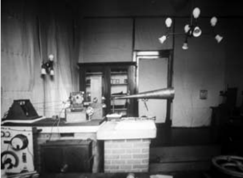
Phonodeik lab with vibration-free platform
